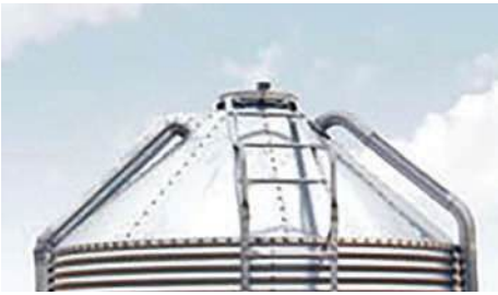
40° roofs provide additional strength and capacity
