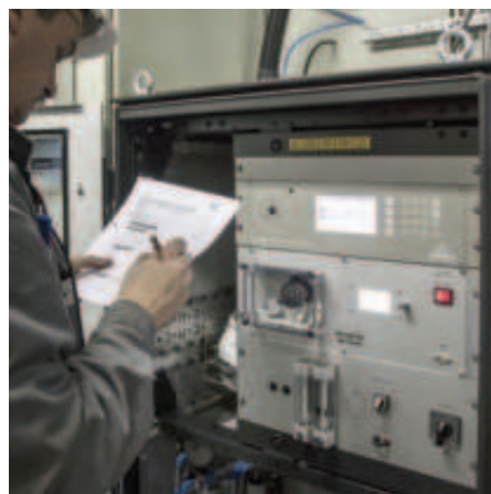
MERCURY DETECTION IN FLUE GASES
