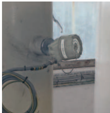
COMPACT SENSOR FOR BROKEN BAG DETECTION
